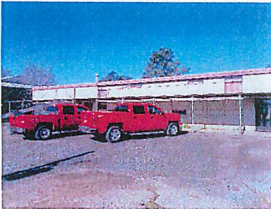
Photo #1 General view of the front of the cafeteria building.
