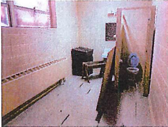
Photo #9 General view of the restrooms behind the stage.
