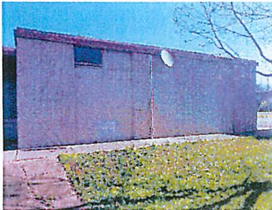
Photo #3 General view of the left side of the cafeteria building.
