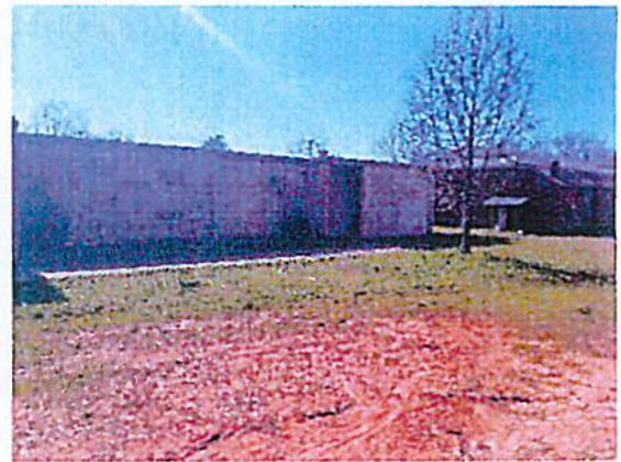
Photo #4 General view of the rear of the cafeteria building.
