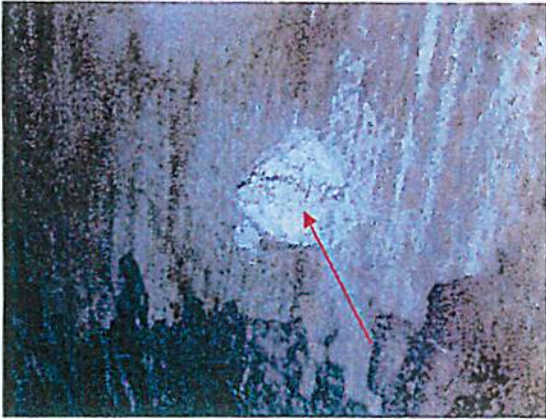
Photo #25 View of boiler body insulation (HA-K) on the boiler.
