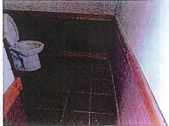
Photo #8 General view of the restrooms next to the kitchen.
