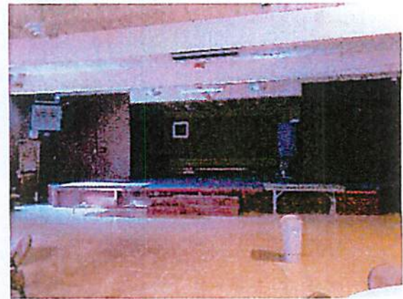
Photo #6 General view of the stage area of the building.
