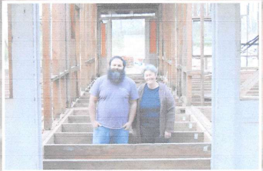
CAITLIN HERRINGTON FOR THE JOURNAL Nick Gambrell and Carla Honea stand inside the partially disassembled Bearden-Gambrell farmhouse. The pair has been working full-time since July to label, sketch and photograph each and every piece of the house in order to reassemble the home.
