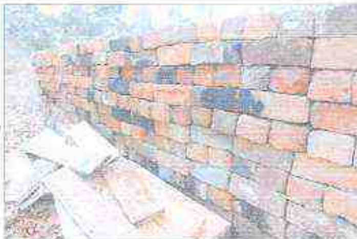
Every brick from the three chimneys of the Bessie Campbell house was removed by hand and stacked on-site, including the bricks taken from the exact opposite order of deconstruction, according to Rick Campbell.
