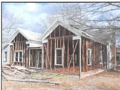
A rear view of the house shows the framework during disassembly.
