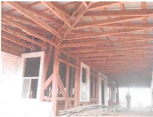
Sample image of house being disassembled
