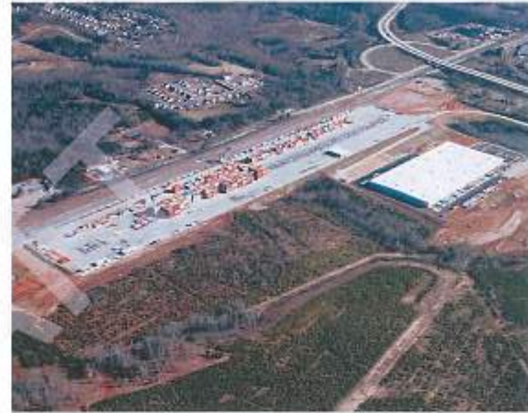
An aerial view of the Greer Inland Port. Photo credit: The SC Ports Authority.
