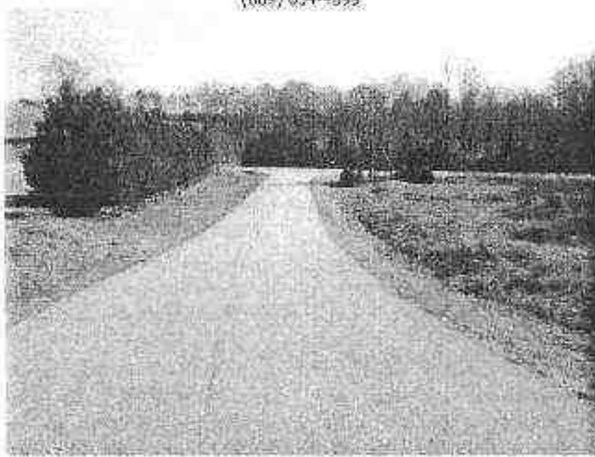
Photo 3. Twin View Drive looking back towards Critter Road.
