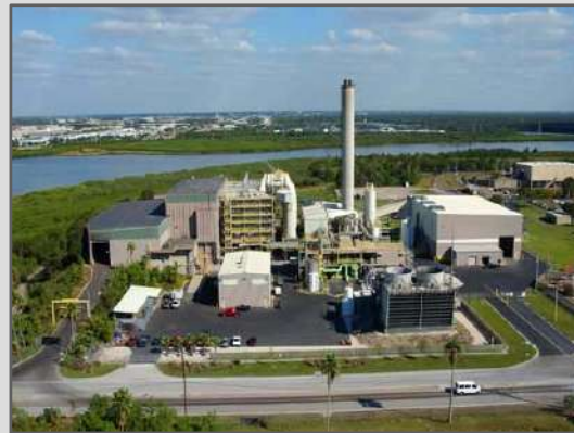
McKay Bay Refuse-to-Energy Facility (Photo Credit: City of Tampa)
