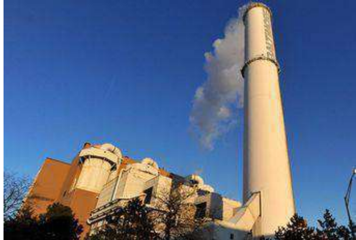
Municipal Solid Waste Incinerator in Baltimore, MD (Photo Credit: Baltimore Sun)
