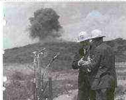
The official groundbreaking on April 11, 1967 for the Keowee-Toxaway Power Project included South Carolina Governor Robert McNair (left) and Duke Power President W.B. McGuire (right) detonating a dynamite blast.
