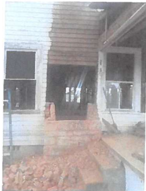
This photo shows the lower section of one chimney. All three chimneys have a granite base and firebox inside.
