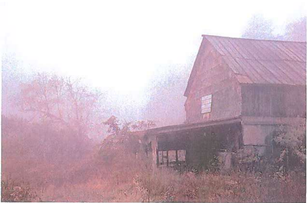
The plan for the property is to remove the dilapidated structures on the property, remove the non-native fishes and the dam to then restore the flow of Pig Pen Branch.
