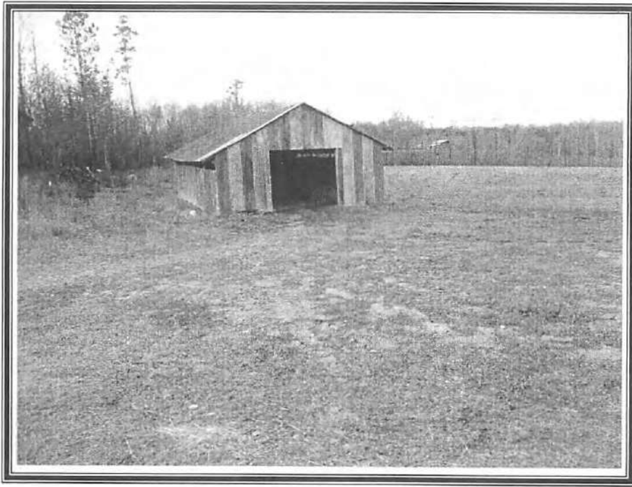
View of barn structure
