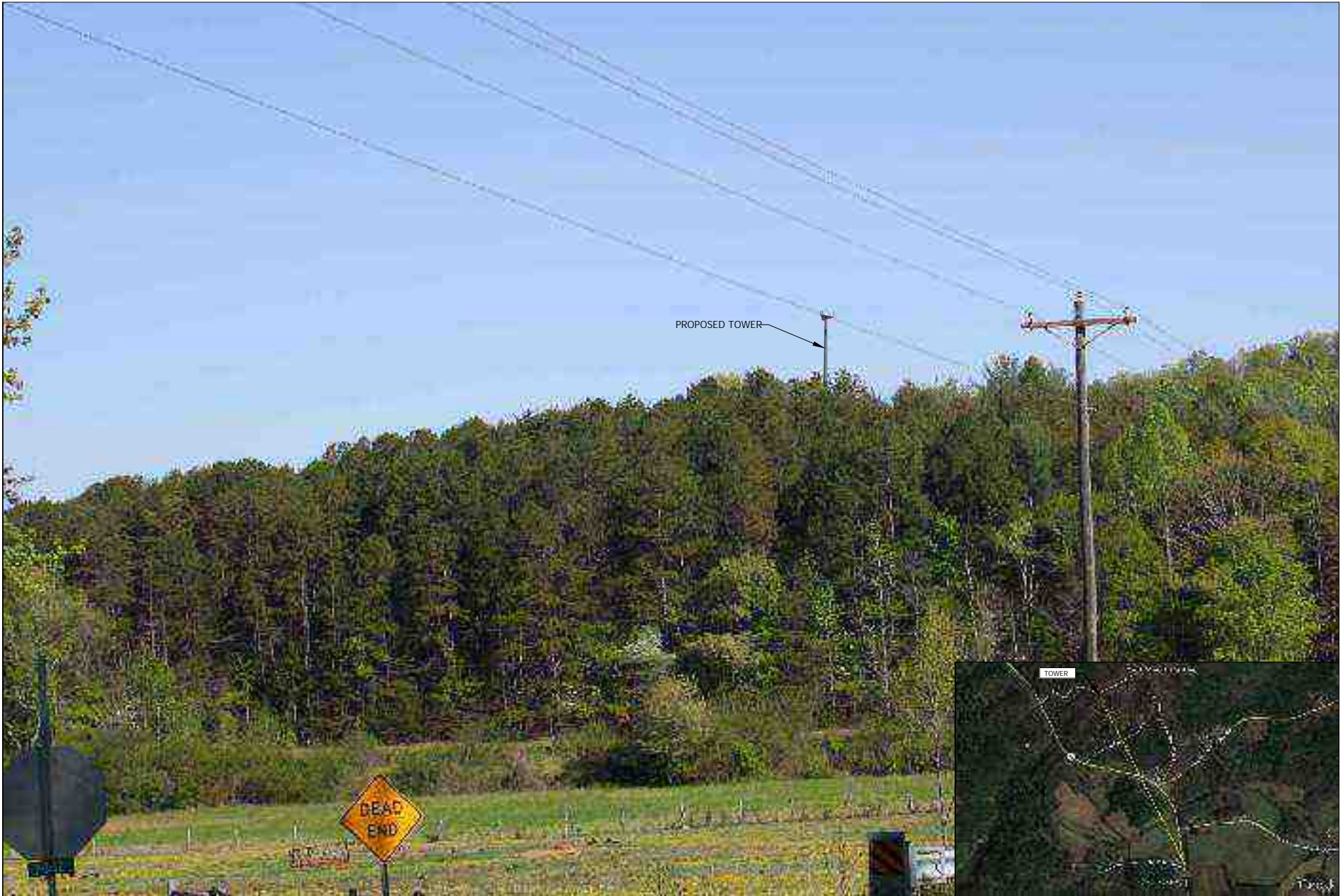
LONG CREEK HIGHWAY AND HUNICUTT DRIVE, LOOKING NORTHWEST, 2600' FROM PROPOSED TOWER
