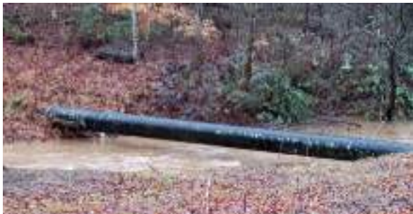
Sewer crossing above Burns Mill Bridge
